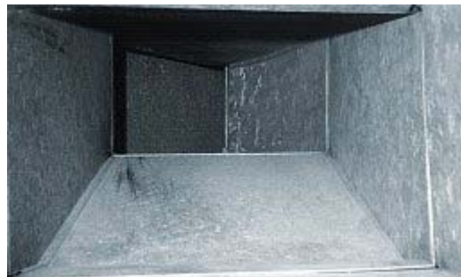
Clean Air Duct after Tri State Cleaning.
